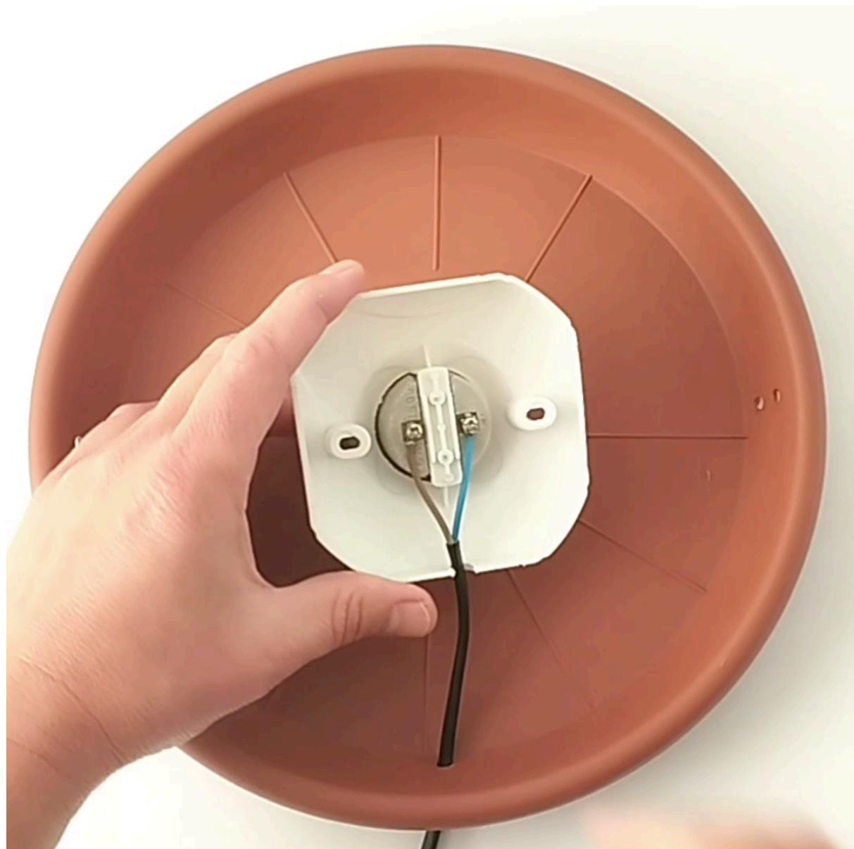
Step 10: Use a 250mm cable tie to attach the bulb holder's base firmly to the plastic saucer, and cut off the excess part.
