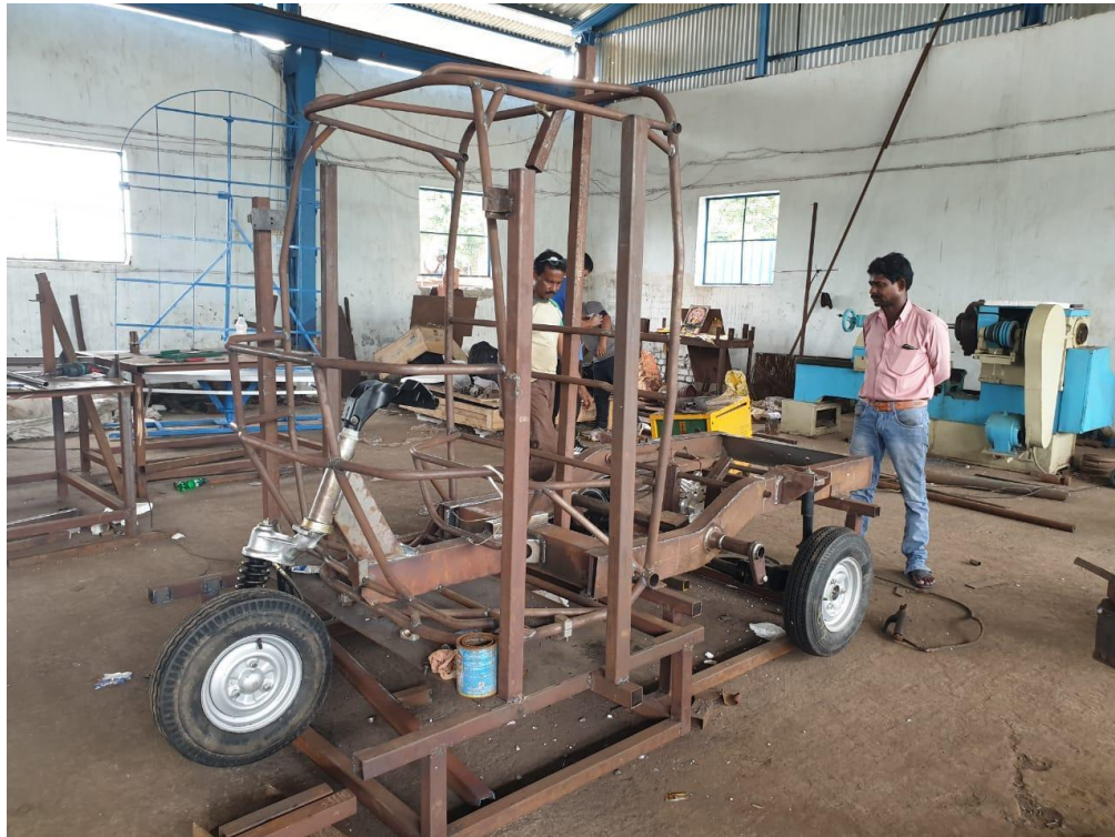
Total Structure Assembly
