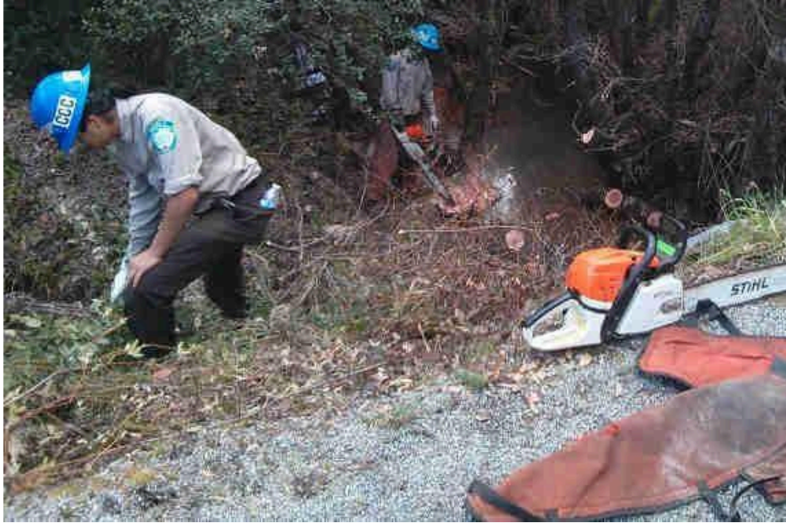
Fig. 5. CCC Crew working along Peters Creek along Portola Heights Rd (after)
