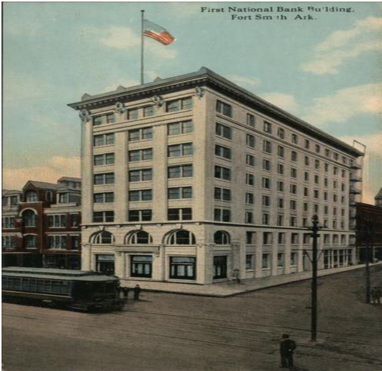
Photo of the Original First National Bank
