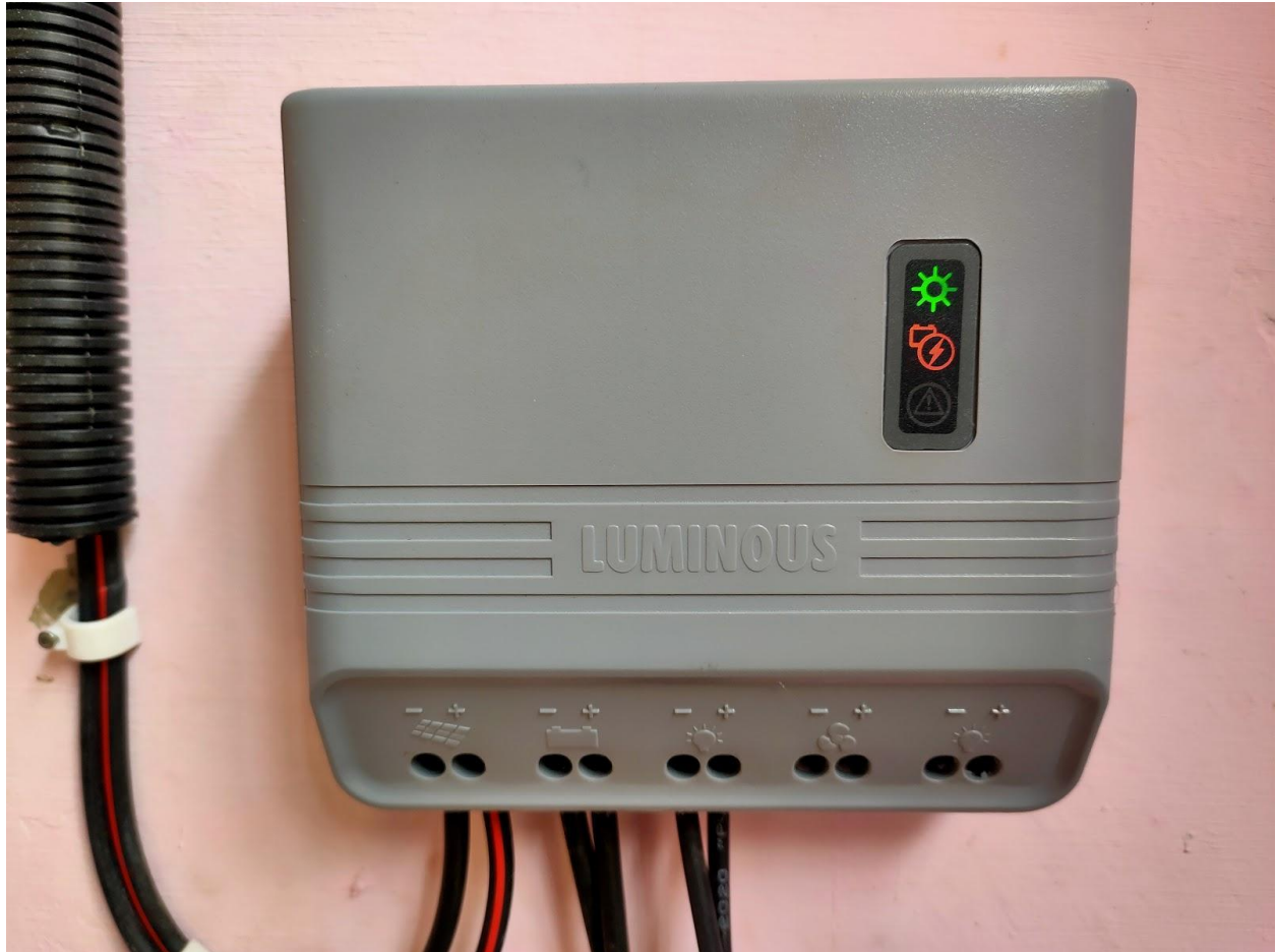
Solar charge controller
