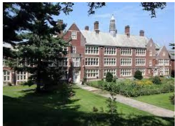
Post Road Entrance
