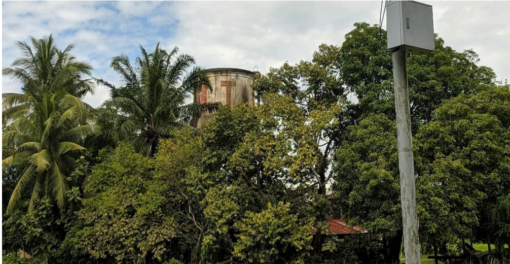
University Water Pumping Station
