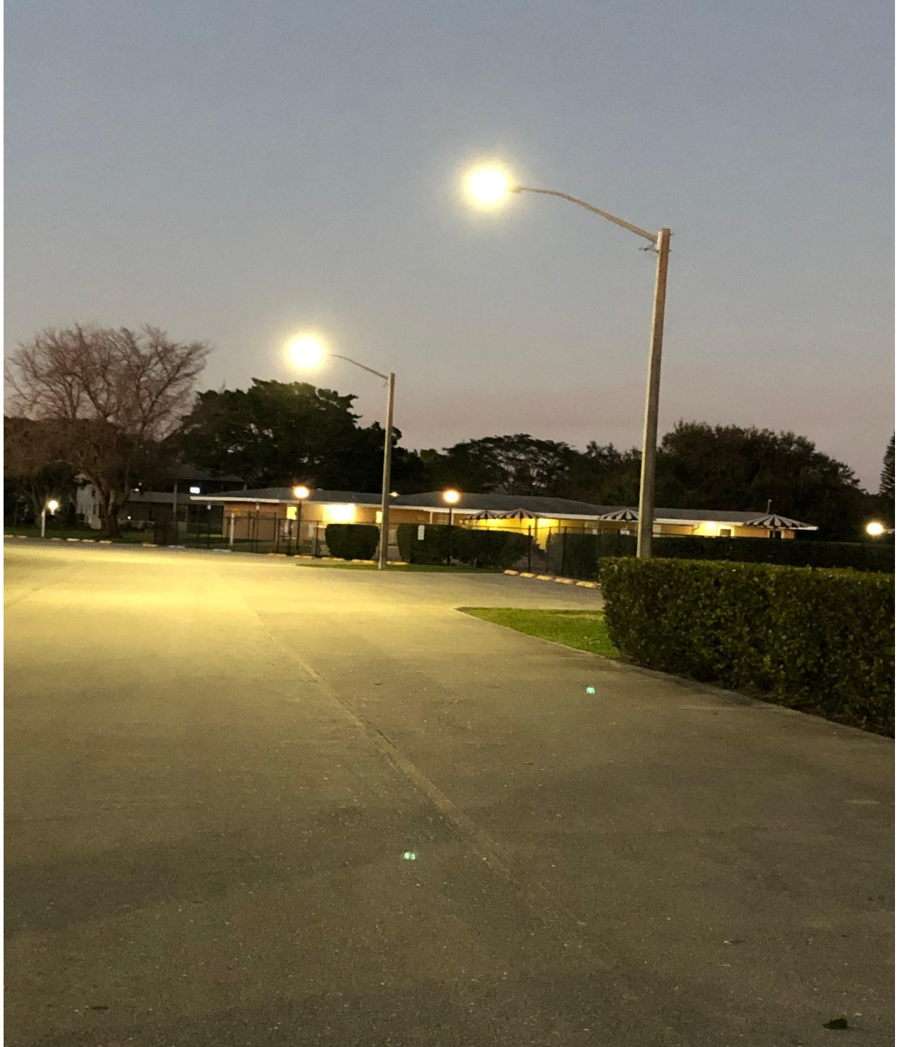
KENT POOL- THESE TWO STREETLIGHTS ARE NOW OPERATIONAL.
