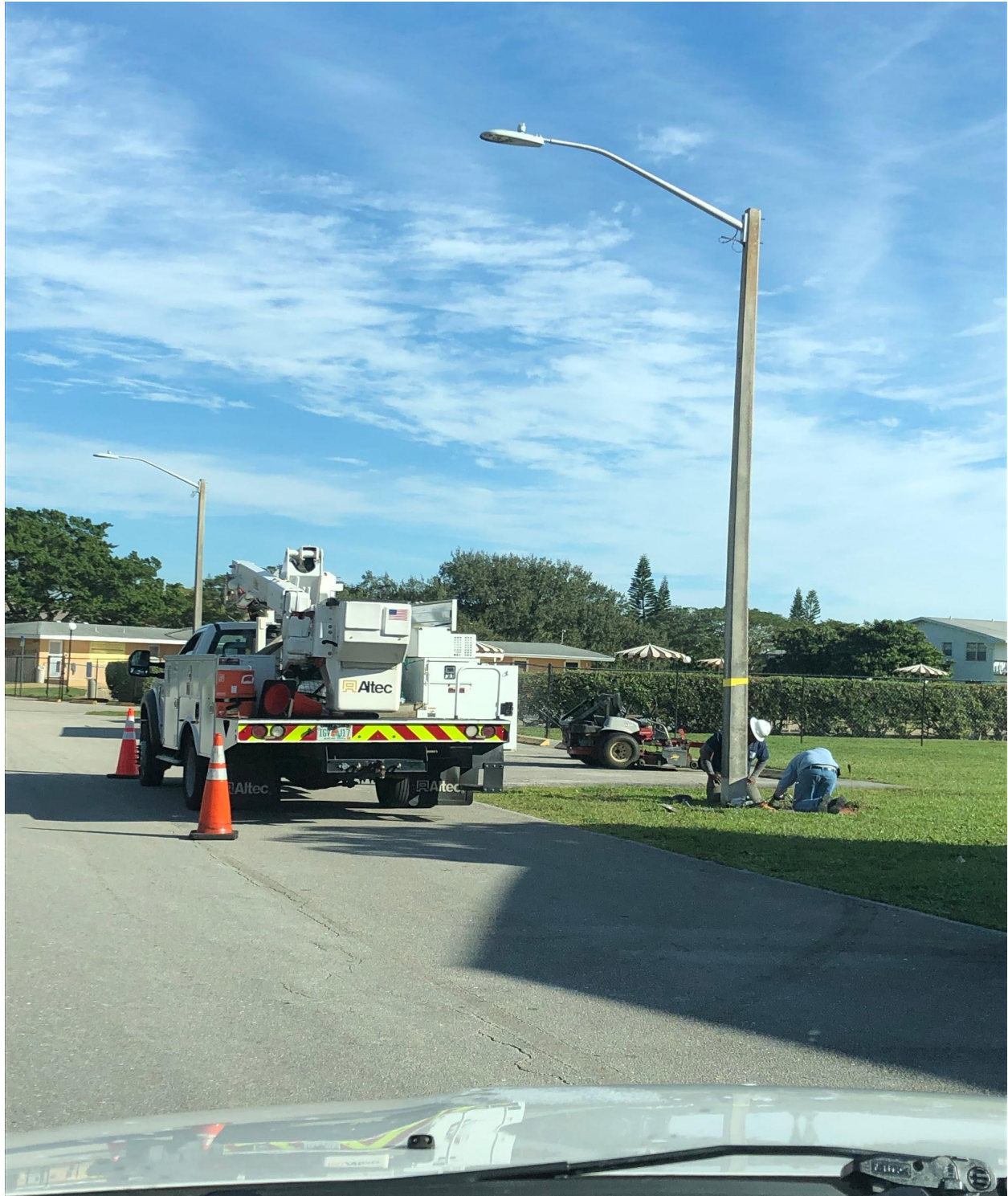
KENT SECTION- FPL FINALLY GOT TO REPAIRING THESE TWO STREETLIGHTS. UNDERGROUND POWER LINES HAD BEEN SEVERED.
