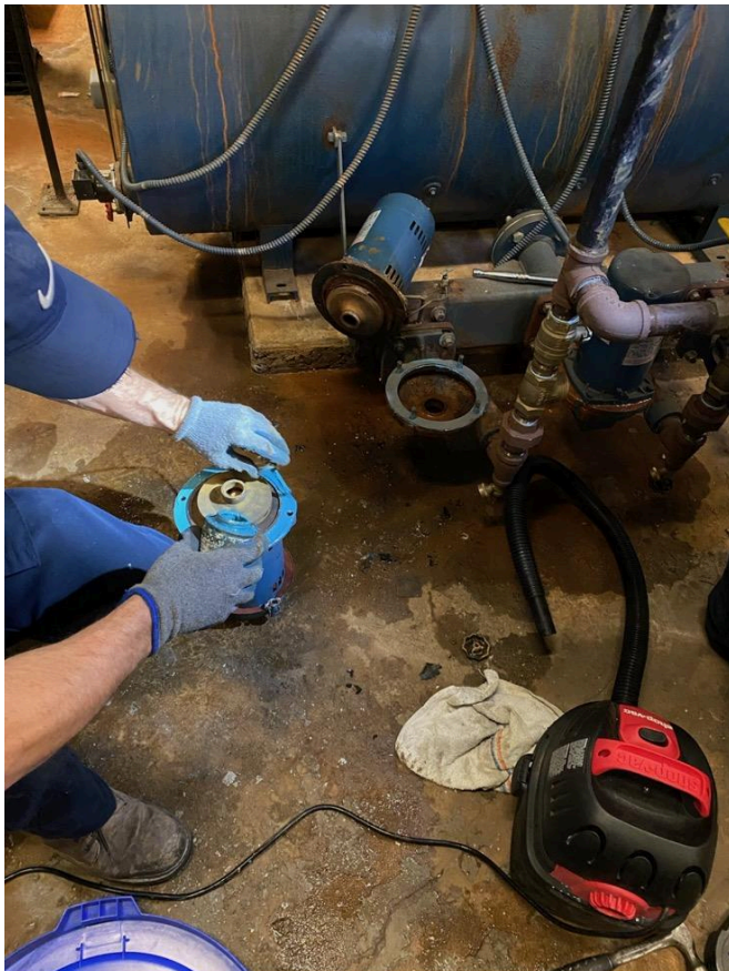
Maintenance was hard at work replacing all three boiler feed pumps and housings at Santapogue. Parts were able to be salvaged from South Bay's old condensate tank that were replaced during this summer's bond project, resulting in significant savings
