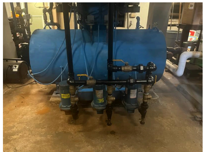
Maintenance was hard at work replacing all three boiler feed pumps and housings at Santapogue. Parts were able to be salvaged from South Bay's old condensate tank that were replaced during this summer's bond project, resulting in significant savings
