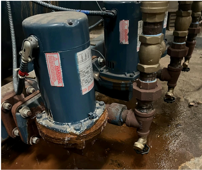
Boiler feed pump housings and bases were corroded and leaking at Santapogue Elementary. Needed to be replaced
