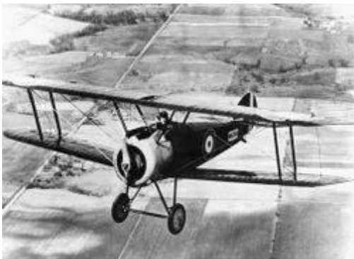
The 1917 Sopwith Camel biplane accounted for more aerial victories than any other allied aeroplane during WWI, destroying over 1,200 enemy in combat. The Camel acquired its name from its two Vickers .303 calibre machine guns, which were housed in a "hump" forward of the pilot.
