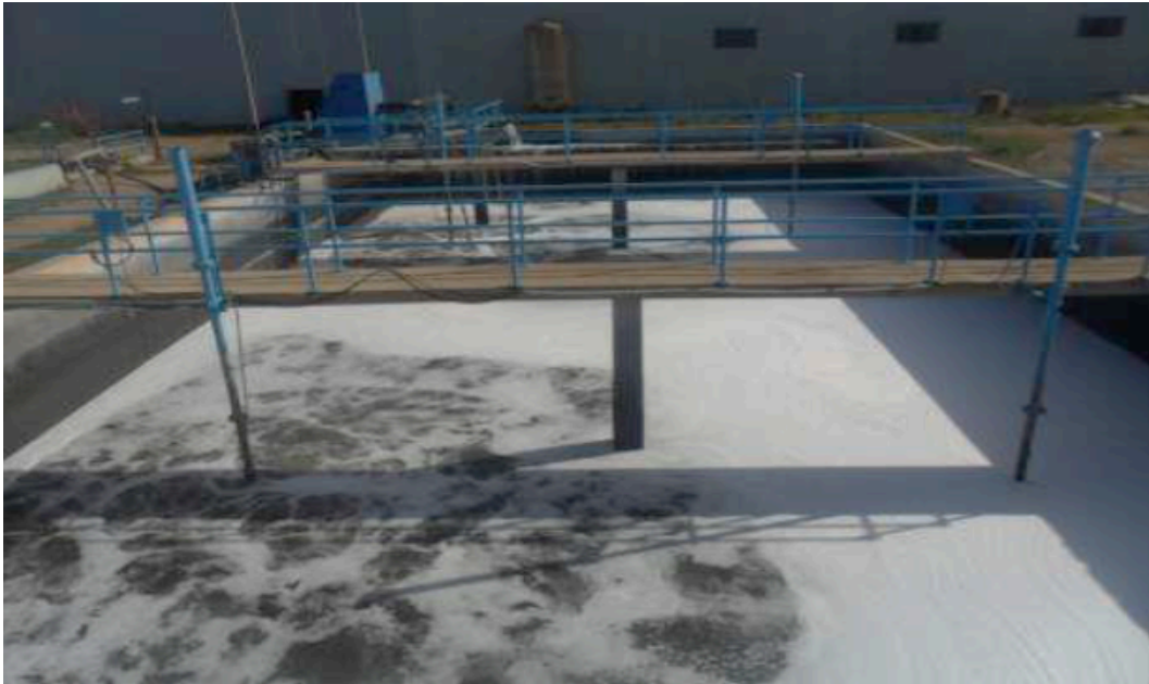
Figure 2. Photo of mixing and equalization basin N ° 1.
