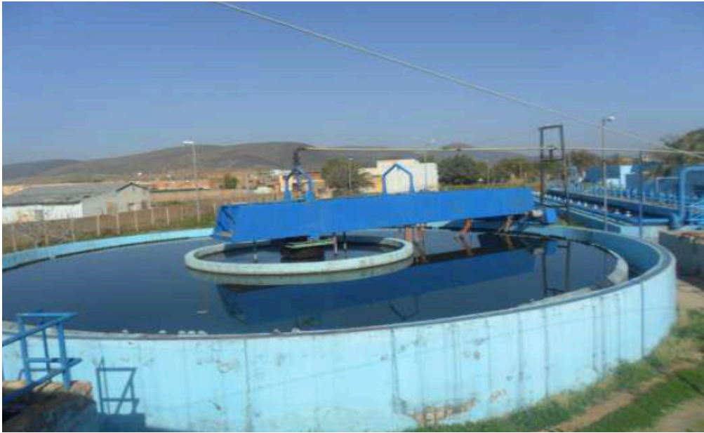
Figure 4. Clarifying flocculator.
