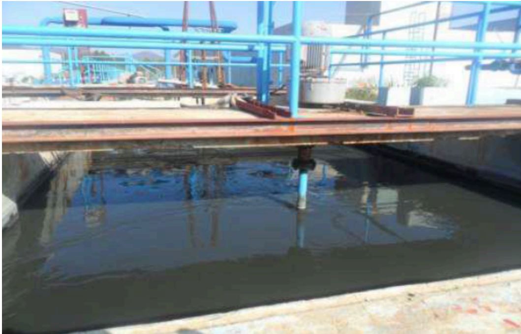
Figure 3. Mixing and neutralization basin N °2.
