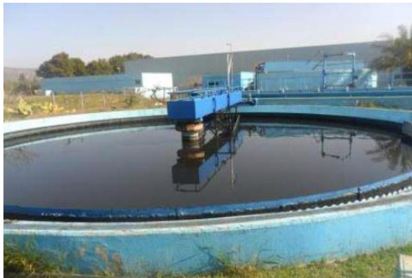
**Figure 6a.** Final clarification basin.
