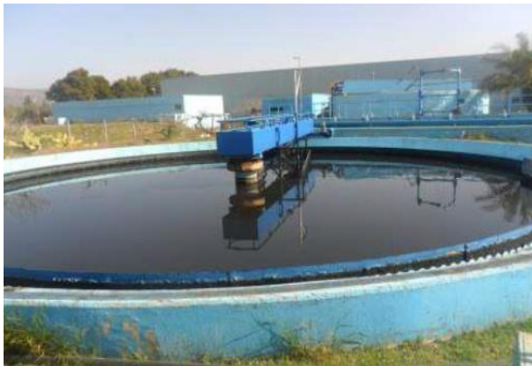
Figure 6a. Final clarification basin.
