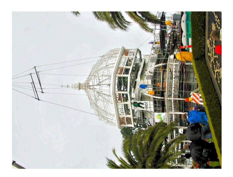
The lifting of the Conservatory dome during its restoration. After major storm damage in 1995 closed the Conservatory, an extensive reconstruction and restoration effort occurred from 2000-2003. Note how the Lowland Tropics was enclosed during this time, allowing plants rooted in place to survive while the Conservatory was reconstructed around them.
