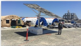
EV ARC™ powering emergency services and medical equipment
