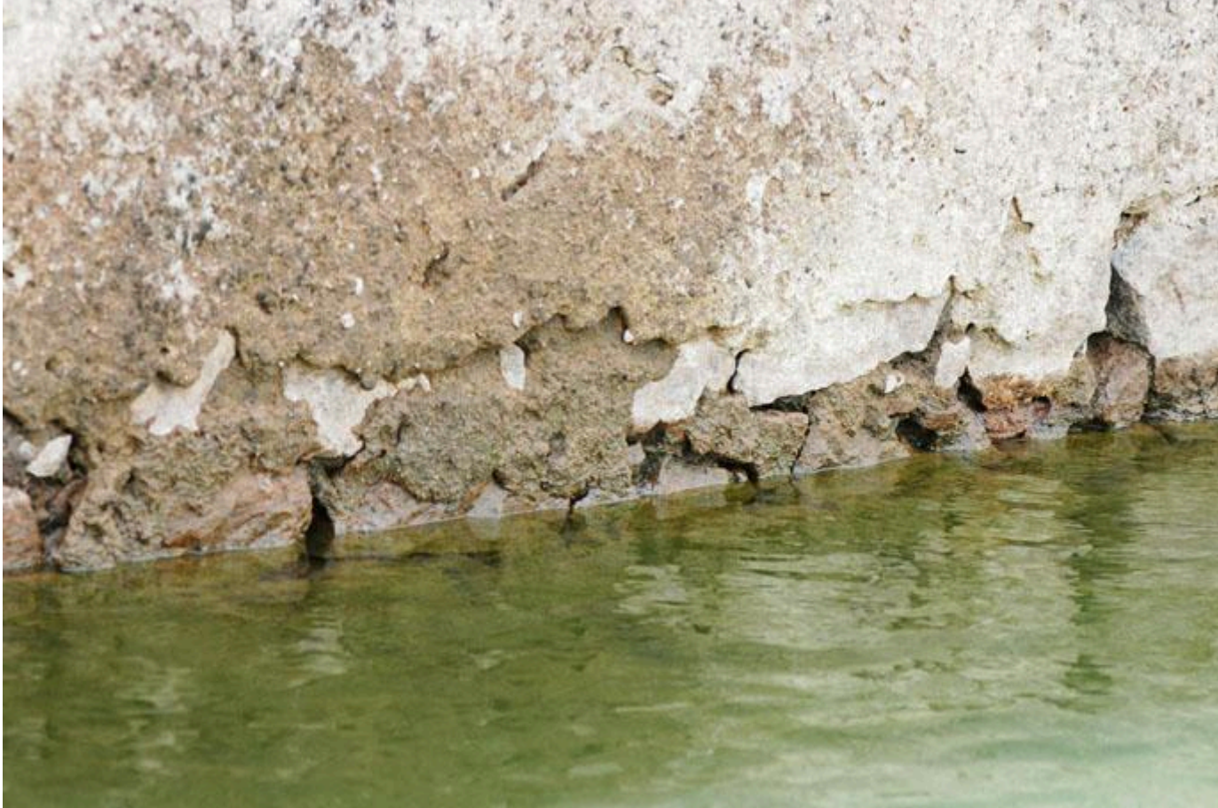
Cracks to the main wall.
