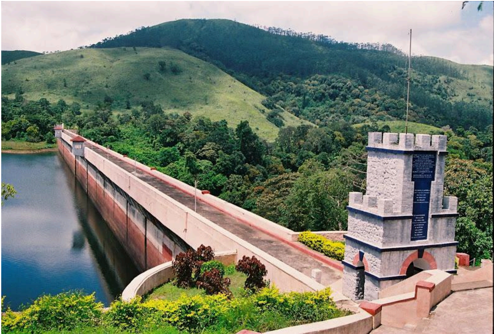
Dam from the top
