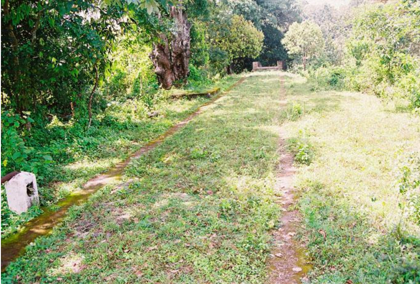
Top of the sand dam between baby dam and main dam.
