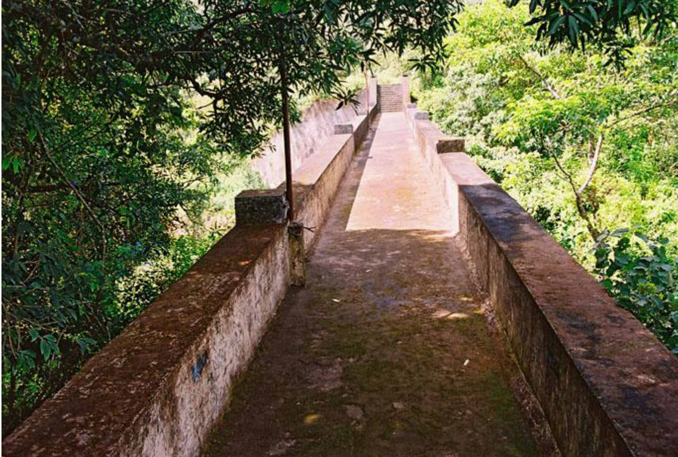
Top of the Baby dam. This is the most weak part in Mullaperiyar Dam.
