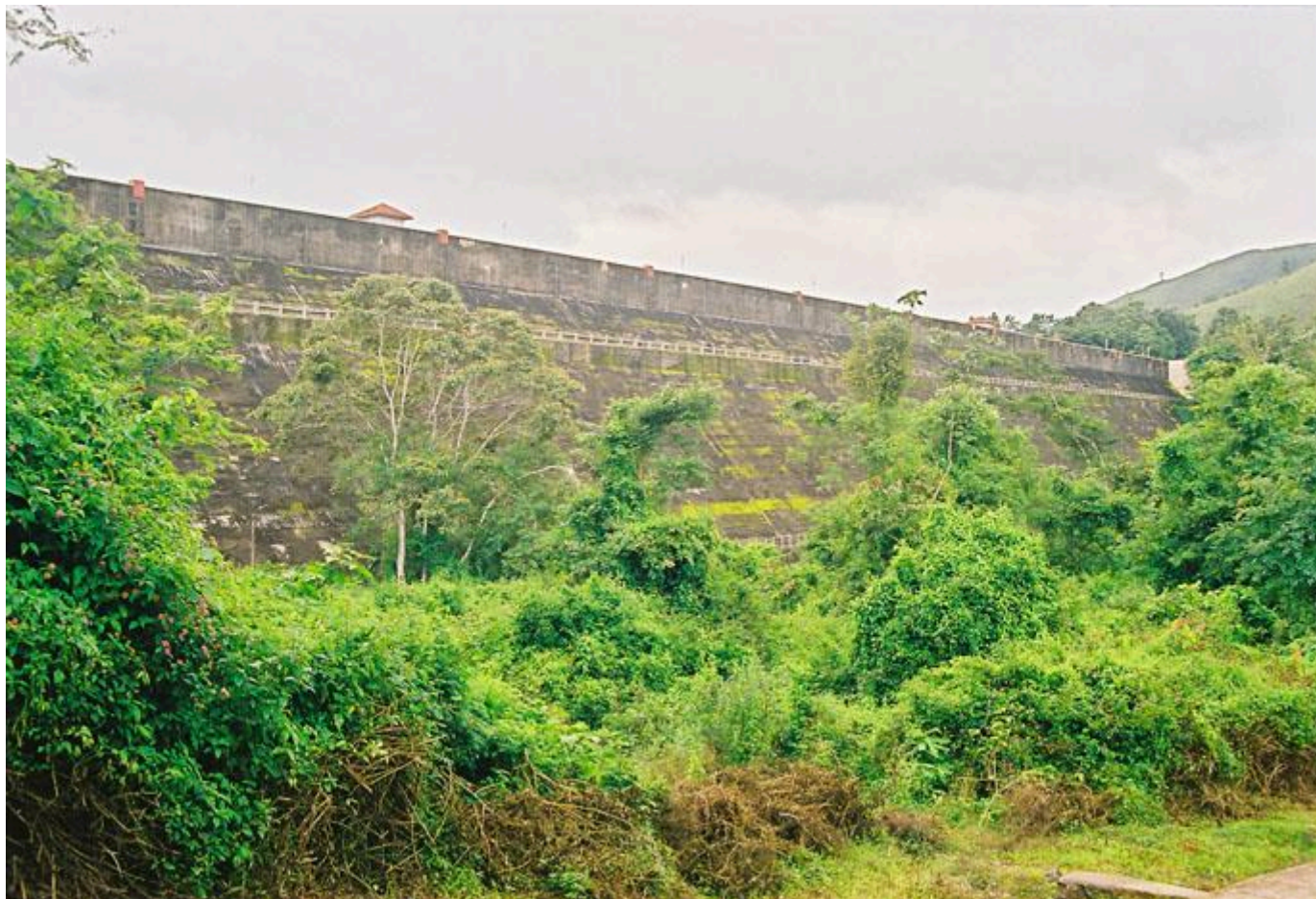
Back side of the Dam.
