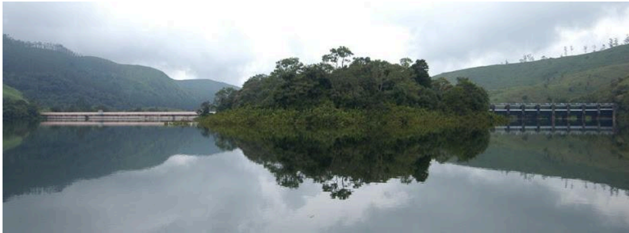
Main dam and spillway
