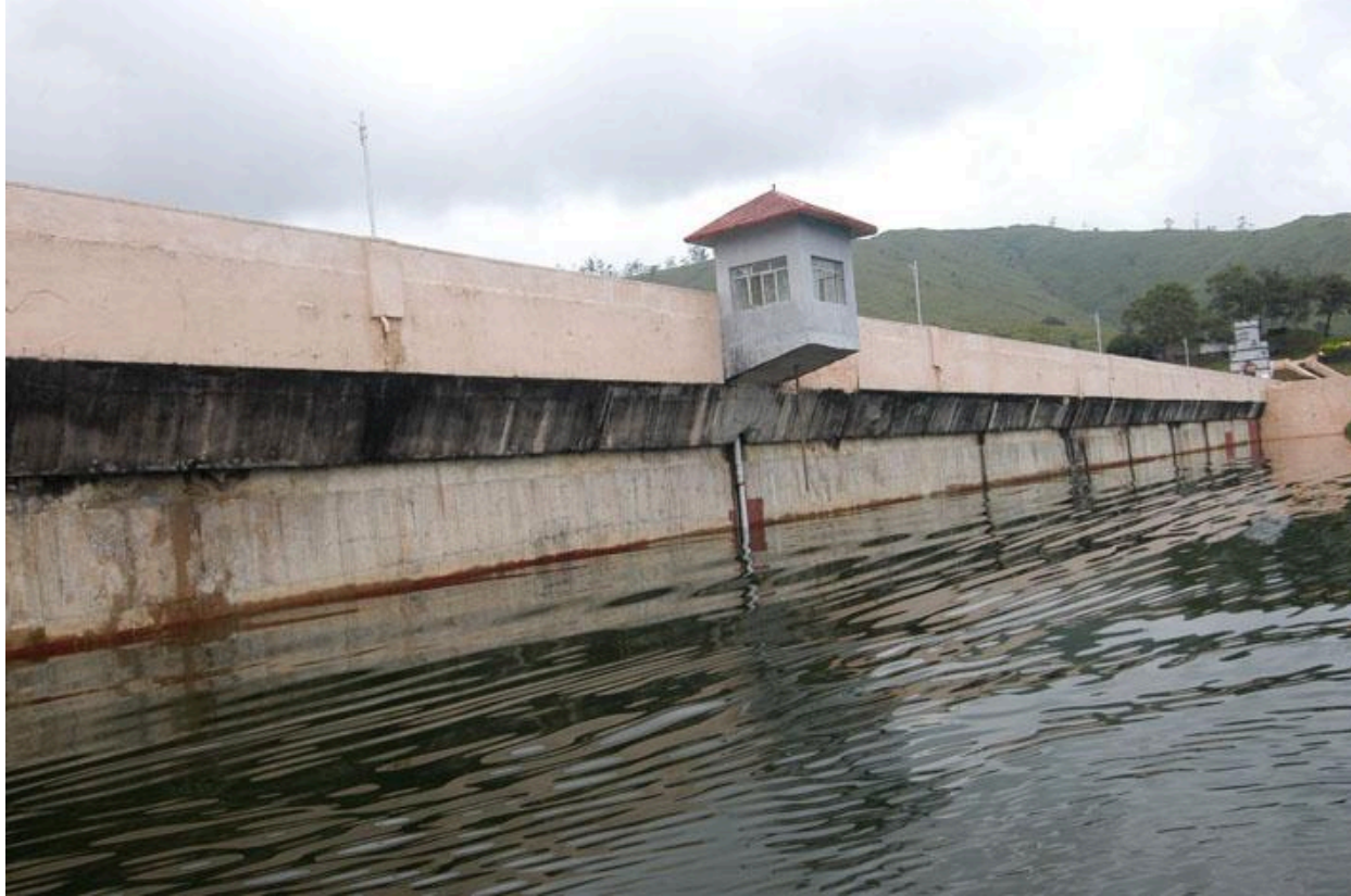
Main Dam view from inside
