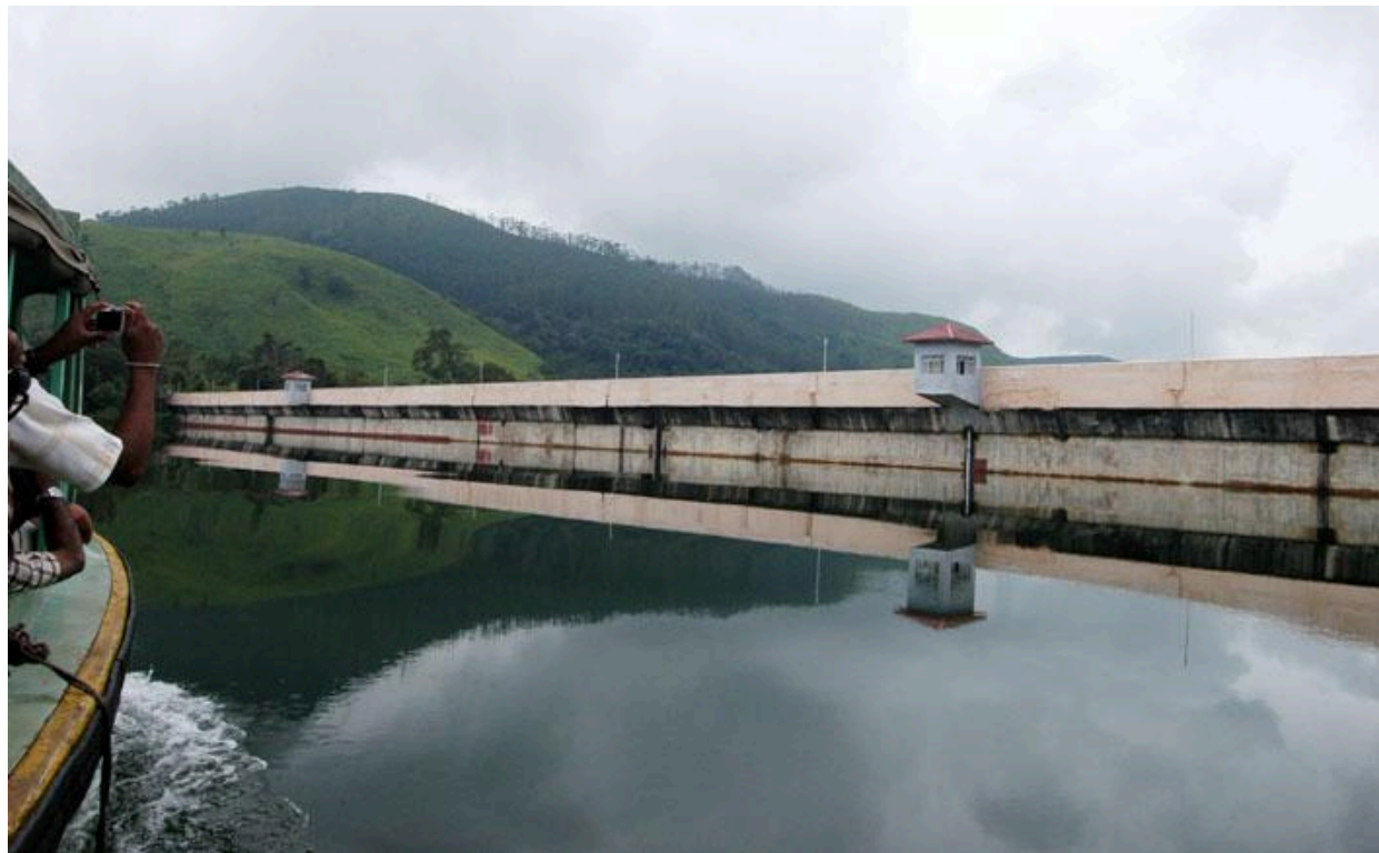
Closer look to the main dam
