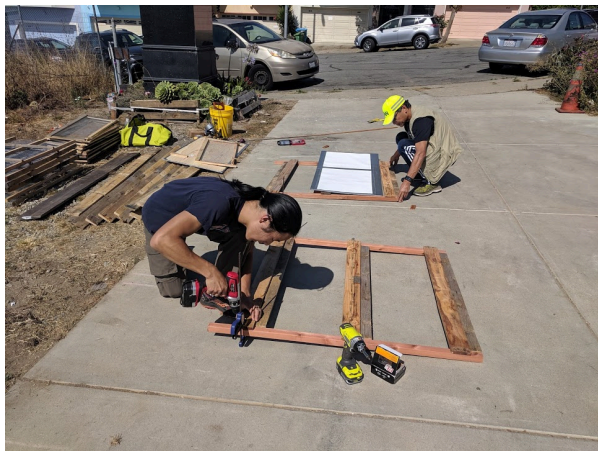
Side modules being assembled with corner posts onsite. In the left of the photo is shown all the other modules yet to be assembled. In picture: Hubert Chen, JD Chen (Dr. Smith, Johnny Chen) Aug 17, 2019
