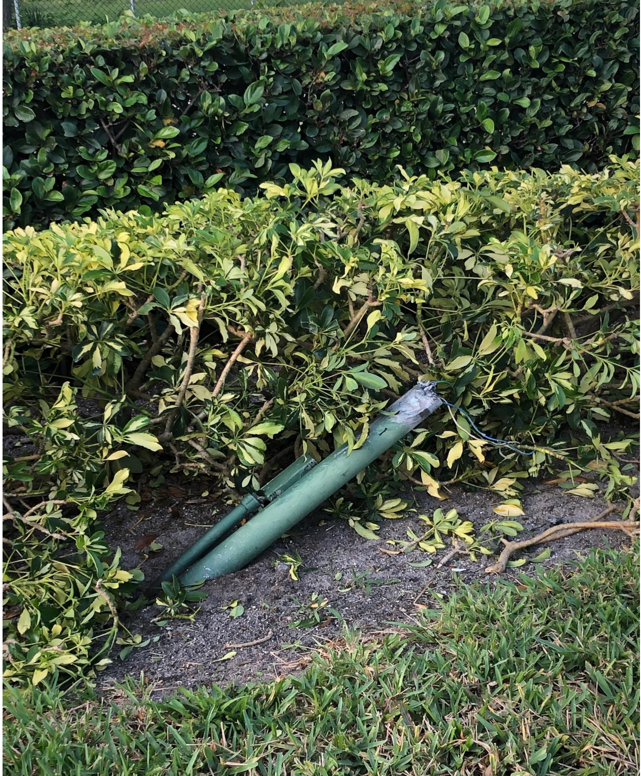
CENTURY BOULEVARD- A VEHICLE RAN UP ONTO A MEDIAN AND DAMAGED SOME SHRUBS AND LANDSCAPE LIGHTING FIXTURES. THESE WILL BE REPAIRED SOON.
