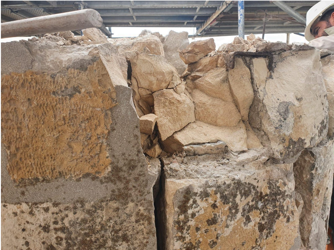
Cracks in the top of the minaret. Credit Ricky Rachman
