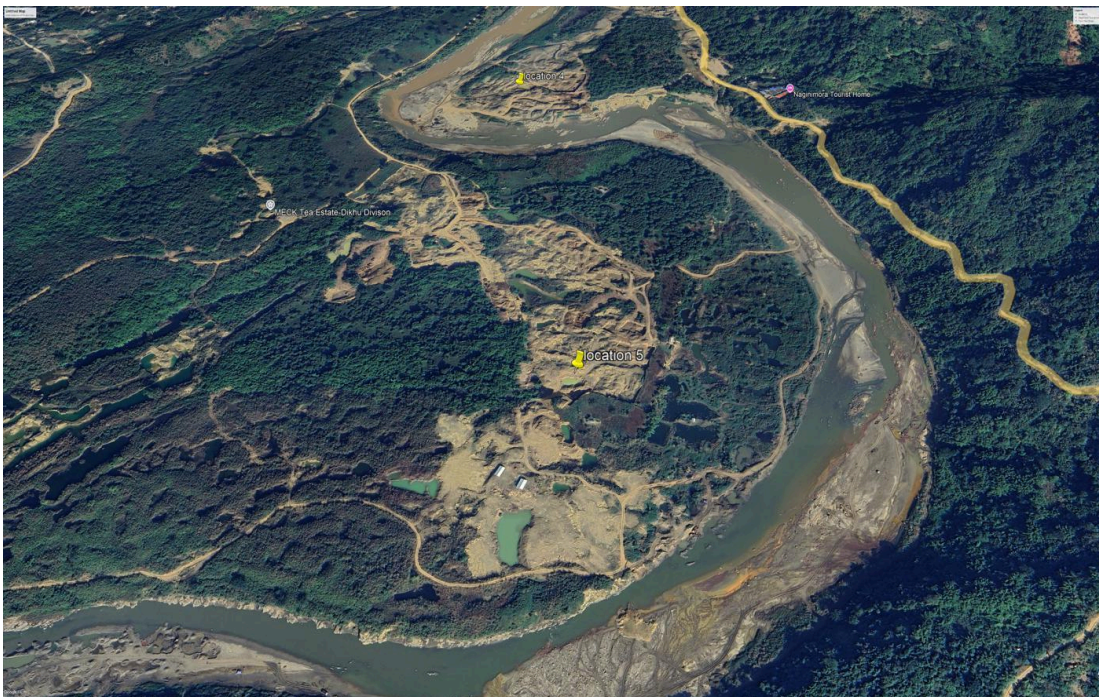
Figure 6b, 2026. The most severe change in the sequence: a large excavation complex with working faces, spoil, settling ponds, haul roads and structures, extending from the bank up onto the hillslope. Bars greatly enlarged; channel choked with sediment; pronounced orange-ochre staining on bar surfaces and along the channel margin downstream of the workings.
