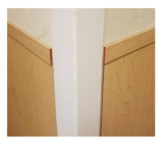
Vertical joints in decorative wall protection materials with any movement must should have a trim covering. A caulk joint cannot handle the movement of the materials.
