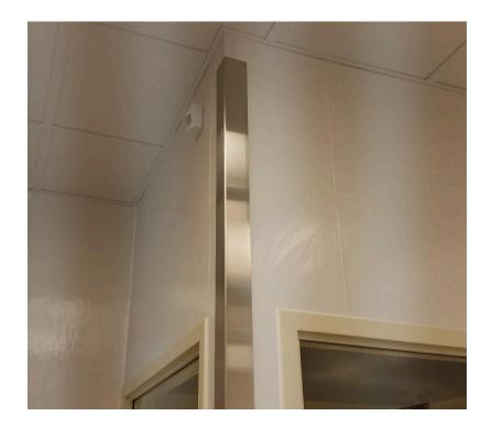
**8. Textured (Pebbled) Fiber Reinforced Plastic sheets** may be used for service corridors, hallways, janitor closets, equipment storage and other back of the house areas. The vertical batten ("T" strip) trim should not be specified as it is easily damaged, and instead a narrow, carefully tooled caulk joint be installed at vertical joints.
