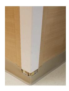
Shock absorbing corner guards on an aluminum retainers tend to slip easily. Below is a bad example
