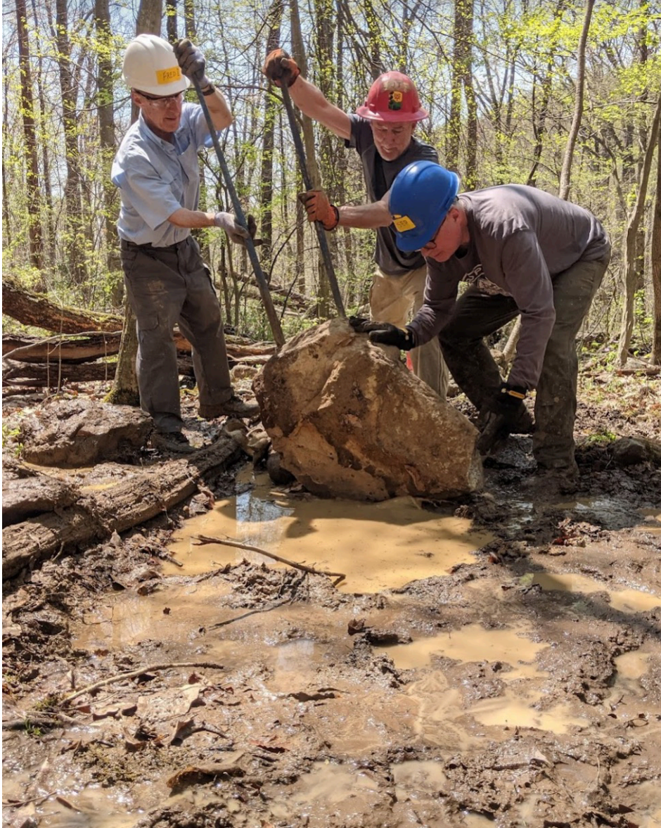
Moving a stepping stone into place. Photo credit Ian Page. Pictured: Fred Meyer, JT Tucker, Steve E. Phillips
