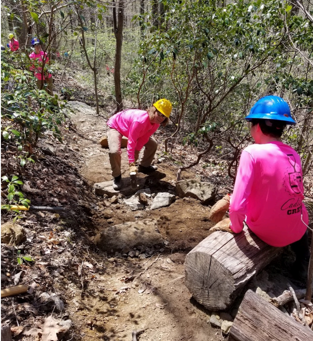
Ellen Shaw making crush as Aiden Badhwar supervises. Photo credit Tysha Robinson.
