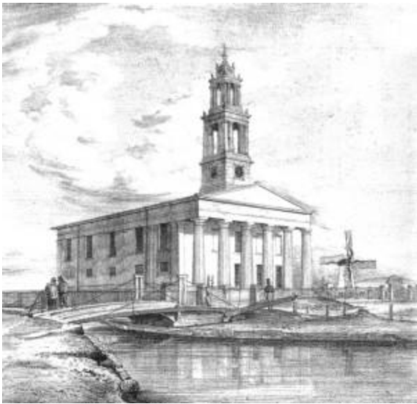
St George's with Wells Way swing bridge and tower mill
