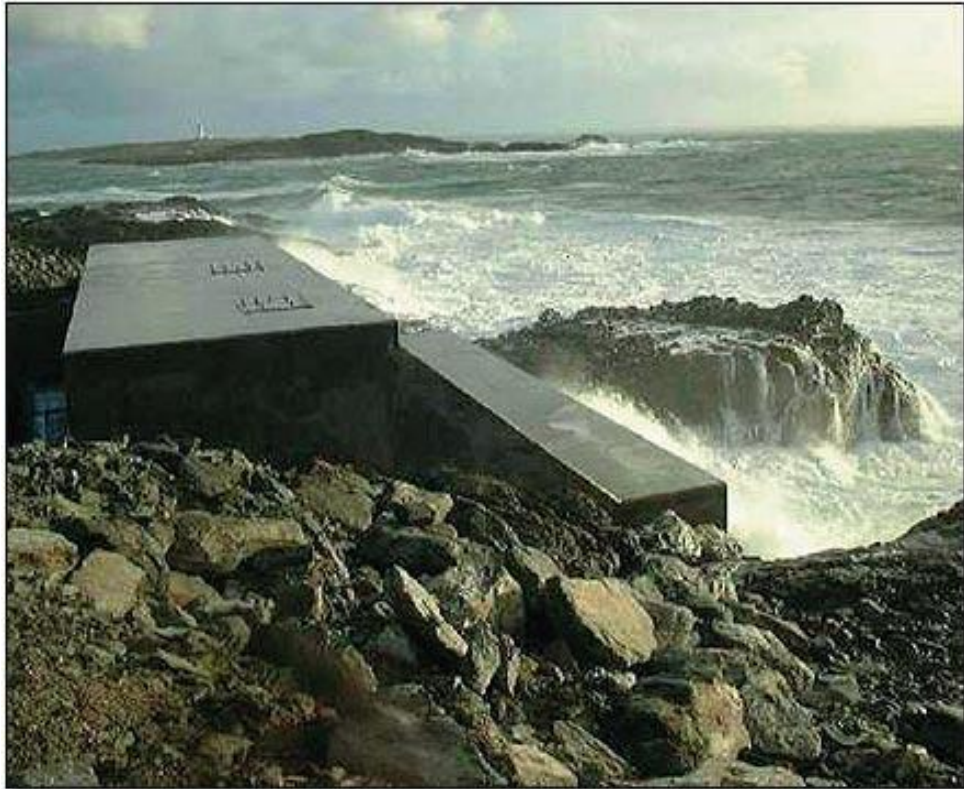
The 500 kW 'Limpet' wave energy plant installed in 2001 on the Scottish island of Islay
