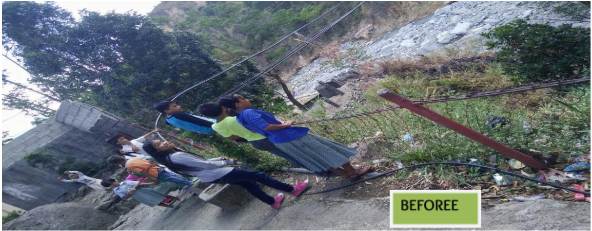
FENCING OF THE SCHOOL PREMISES OF THE CAMP 6 ELEMENTARY SCHOOL
