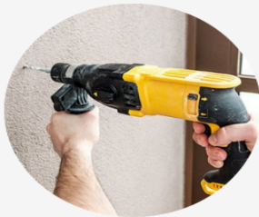
Drilling & Chasing on the Blocks
