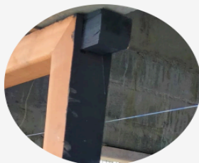
Door Frame Fixing
