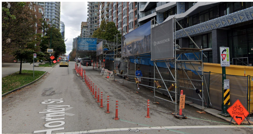
Detour on Hornby Street in the City of Vancouver. Temporary protected lane uses curb stops and delineators to maintain protection from motor vehicles
