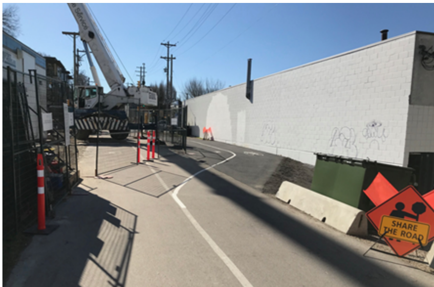
Construction detour implemented along the Arbutus Greenway (City of Vancouver) stays within the greenway right-of-way and maintains the same path quality
