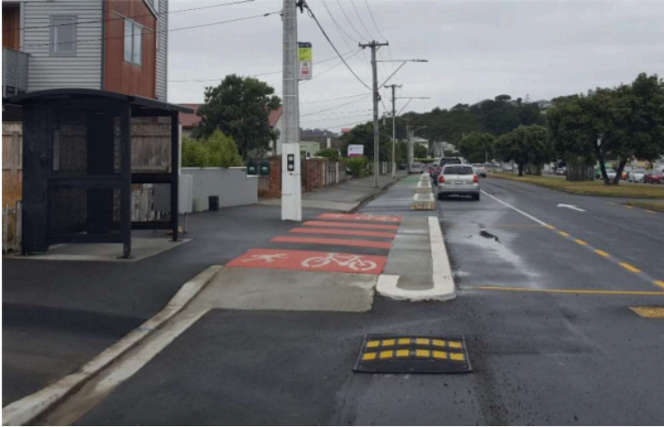
Figure 6: Bus stop bypass where shared zone for cyclists and pedestrians is denoted by red stripes and painted symbols.
