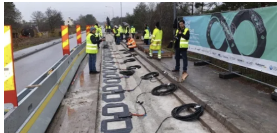
Figure 3.2.2 Transmitter Assembly Layout
