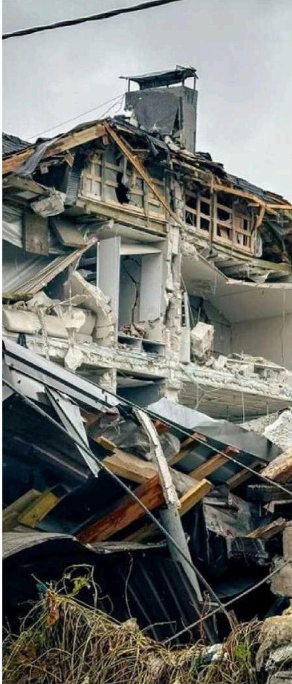
Rice. 12Residential building destroyed by rocket attack
