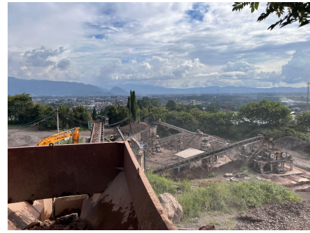
Gambar 1. Tampak keseluruhan unit crushing plant
