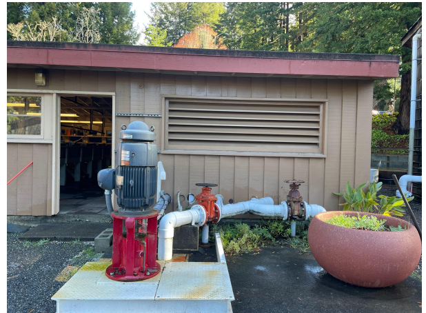
Figure 2. Before and after the installation of the new pump. The new pump allows users to control the speed of the pump, where before the only options were 'on' and 'off'. Users can measure the speed of current flow with a flow meter located inside of the fisheries building.
