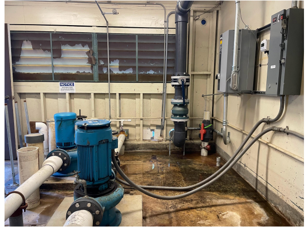
Figure 1. Before and after removal of pumps 1 and 2. Breaker boxes were reduced from 4 to 2, and a digital flow meter was installed. Blue pumps were left as a backup for instances where the new, main pump needs to be shut off.
