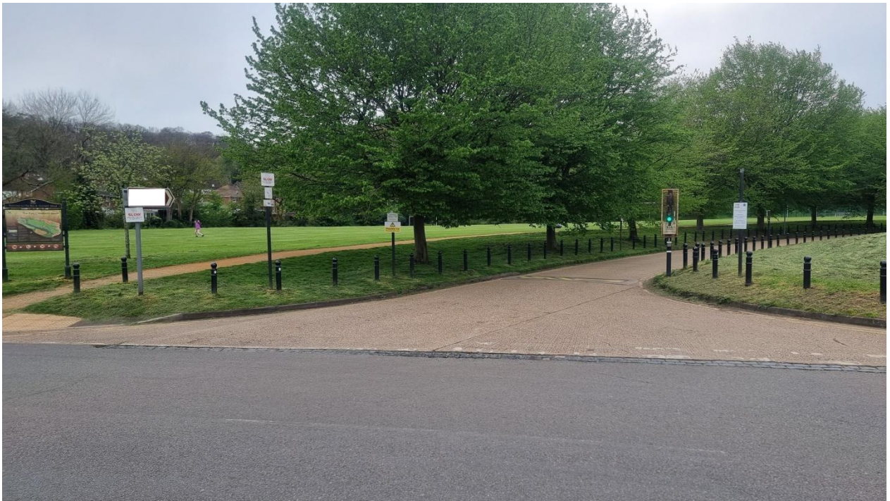
Figure 2: entry/exit of the road leading to [XXXXXX] car park
