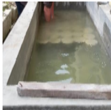
Gambar 4 Perawatan Beton [Times New Roman, 11]
