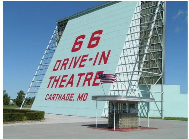
Route 66 Drive In Theater
