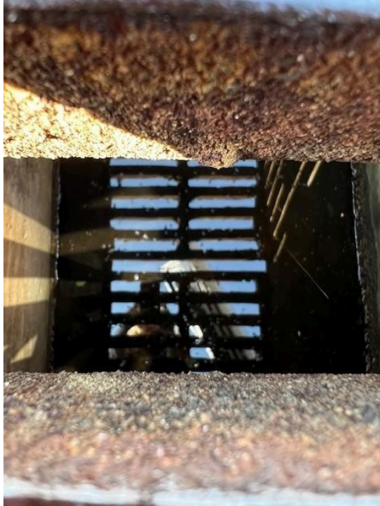
Outfall chamber behind 273 Oak Haven Dr. (some sediment)
