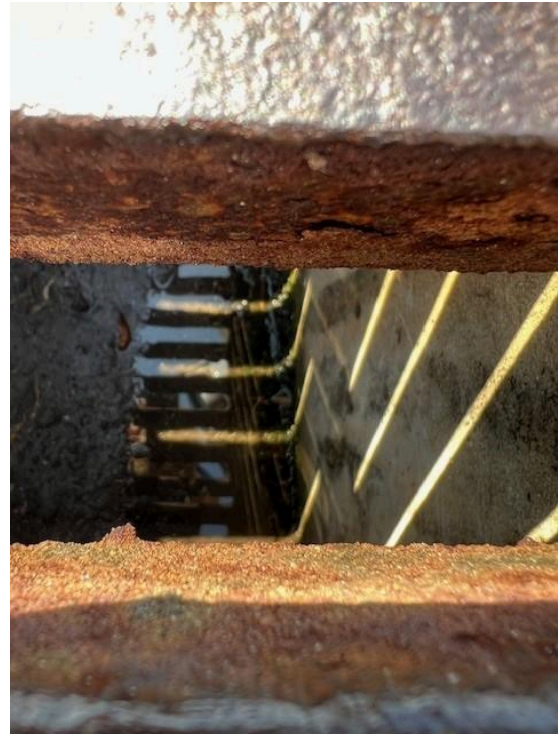
Trench drain (some sediment)
