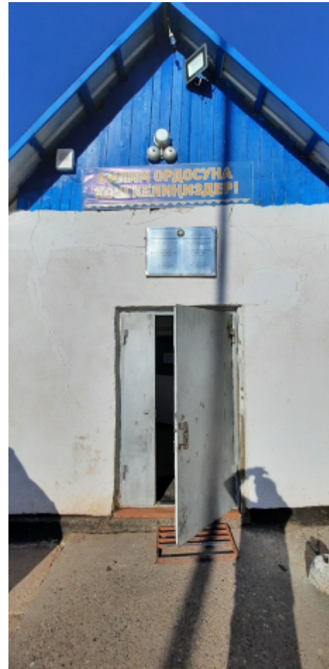
Photos 16, 17. Building No. 1 lacks a ramp for access to the PWD.
