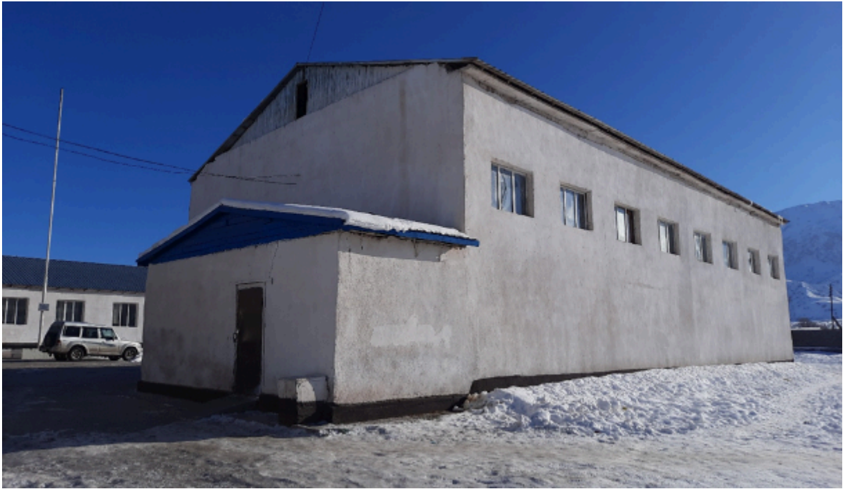
Photo 5. General view of building No. 2 (sports hall) from the northwest side
