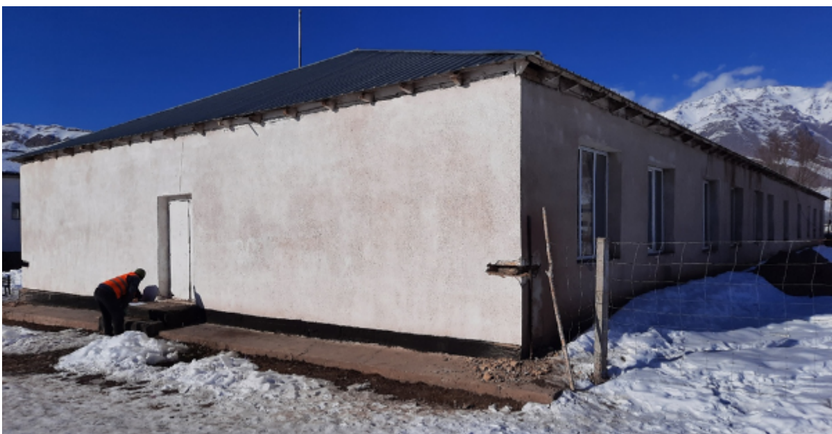
Photo 2. General view of block No. 1-1 from the southeast side
