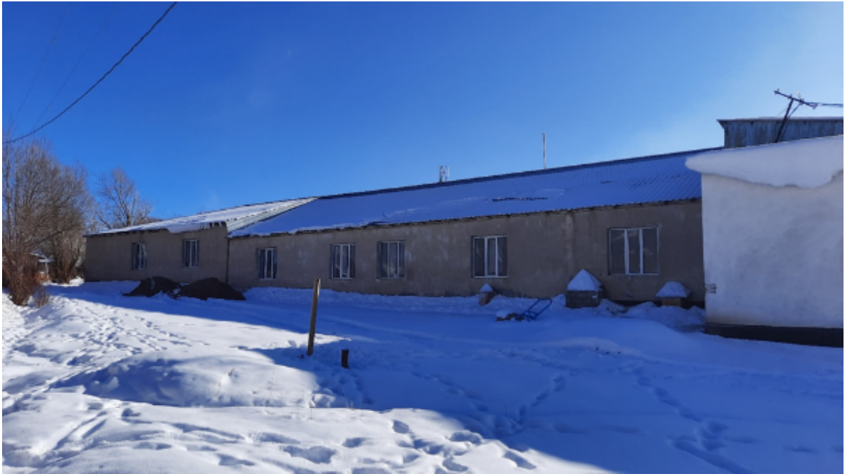
Photo 3. General view of block No. 1-2 from the north side
