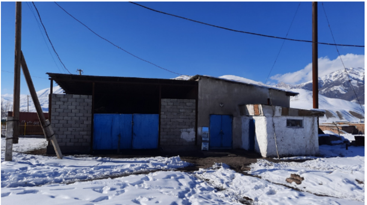
Photo 6. General view of the boiler room from the east side
