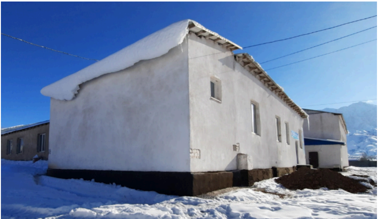
Photo 4. General view of sides 1-3 from the northwest
