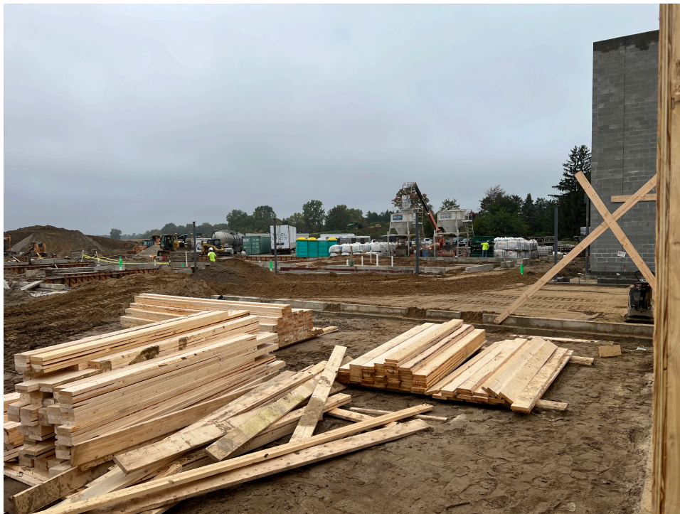
Main Office and Main Entrance
