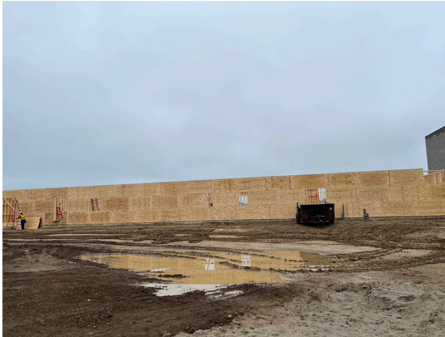
Upper Elementary Wing, Outside Wall
