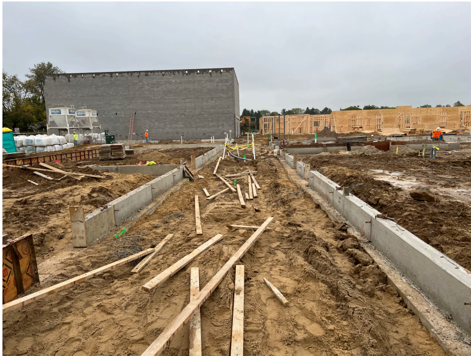
Central Main Corridor
