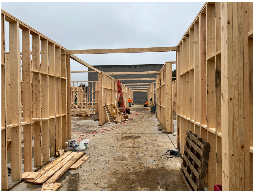
Upper Elementary Wing Interior Hallway
