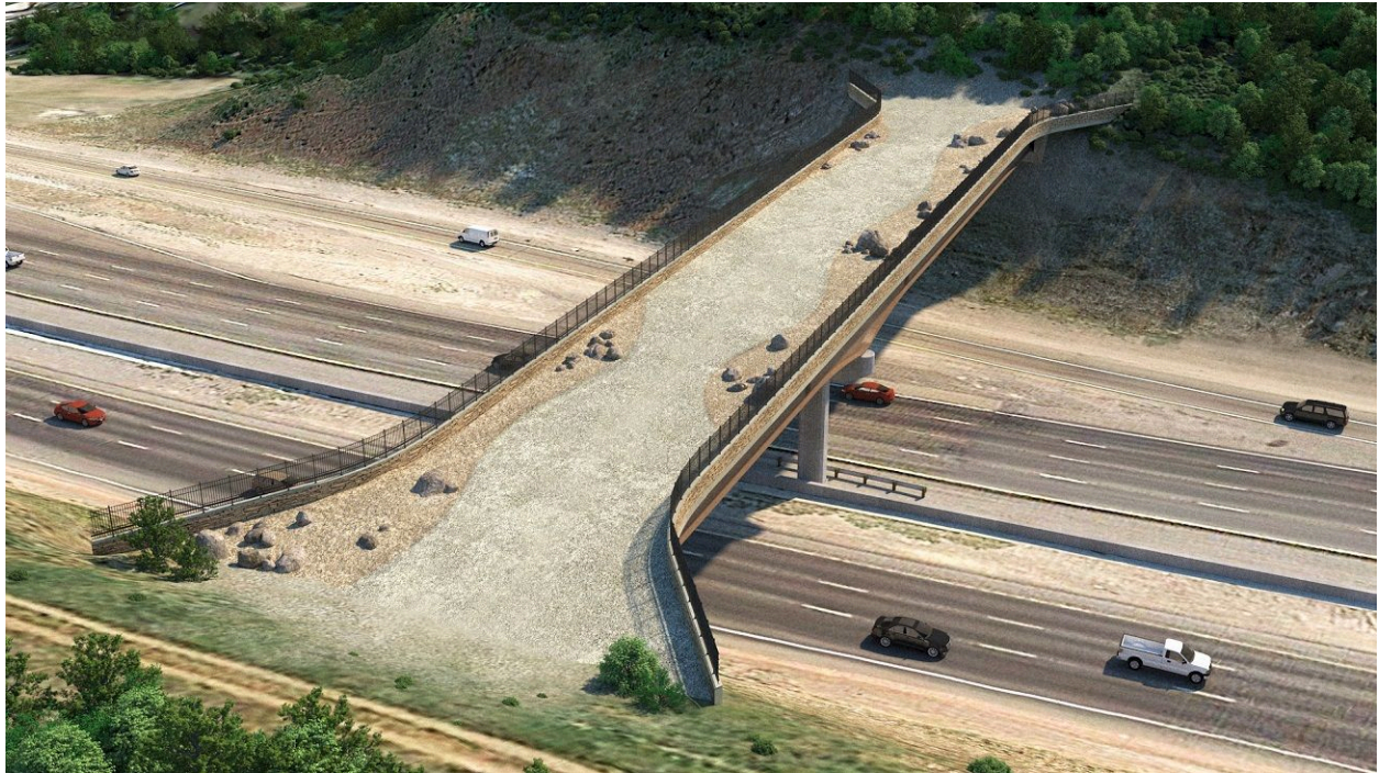
Wildlife bridge construction in progress (Source: WSP)
