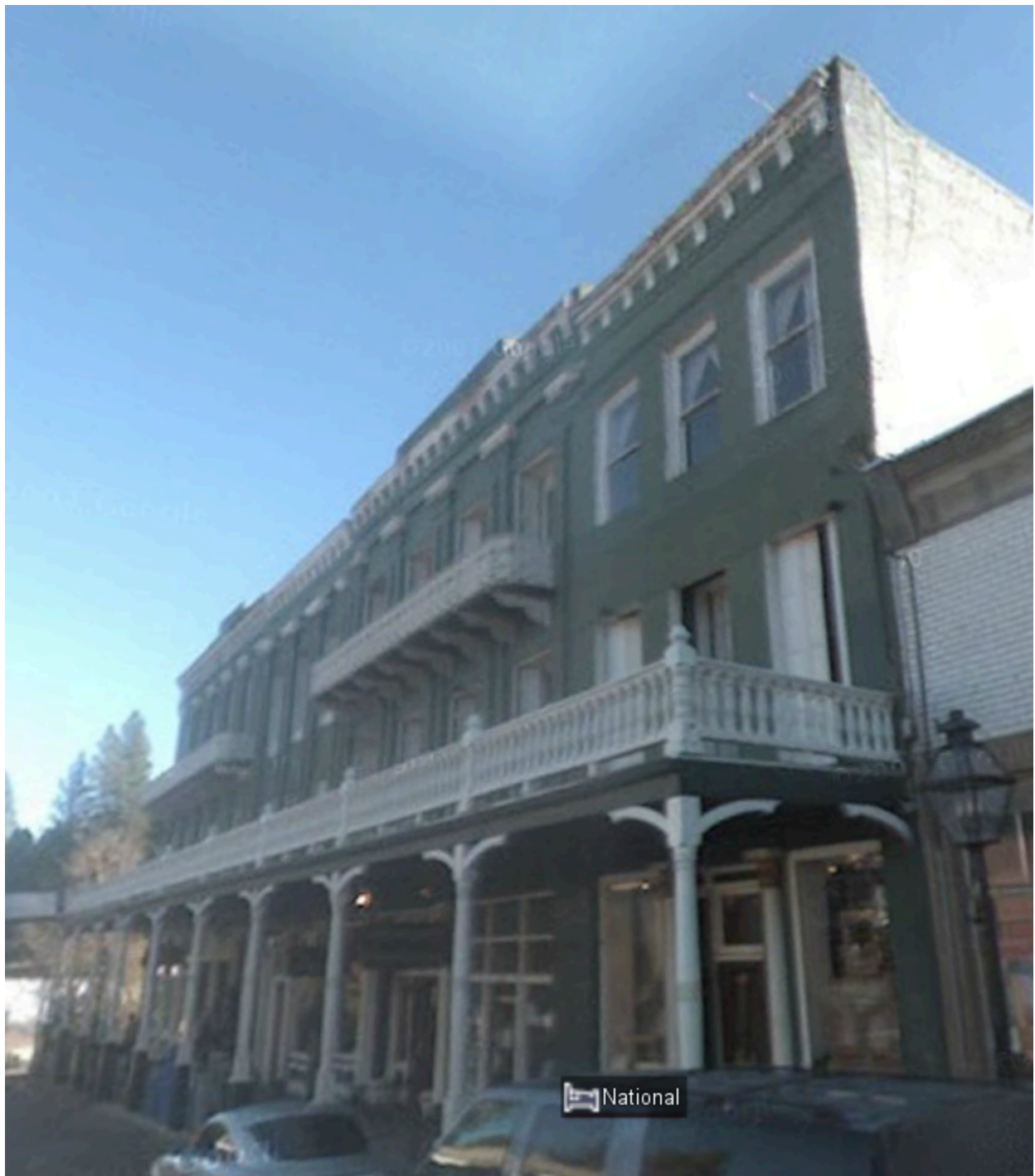
214 Broad Street, Nevada City, California
