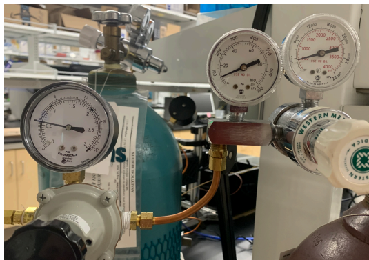
Fig. C9. High and low pressure regulators on the gas tank.
