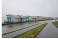
Living with water - not keeping it out Amphibious houses function with different water levels (Maasbommel, the Netherlands)
