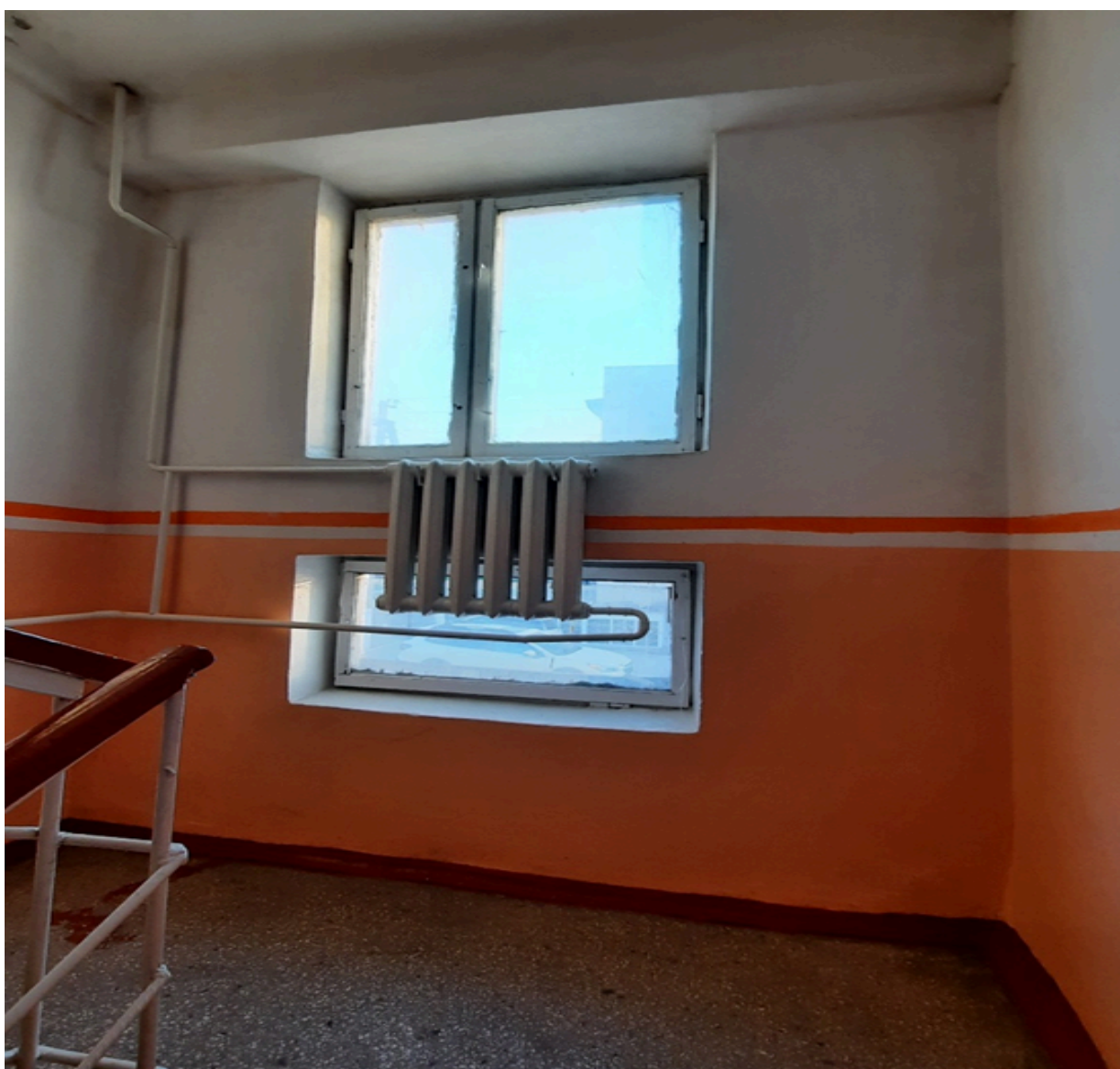
Photo 4. Type of radiators installed in building No. 2. MS-90 cast iron radiators.
