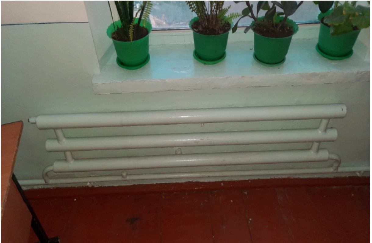
Photo 5. Homemade tubular radiators installed in building No. 1
