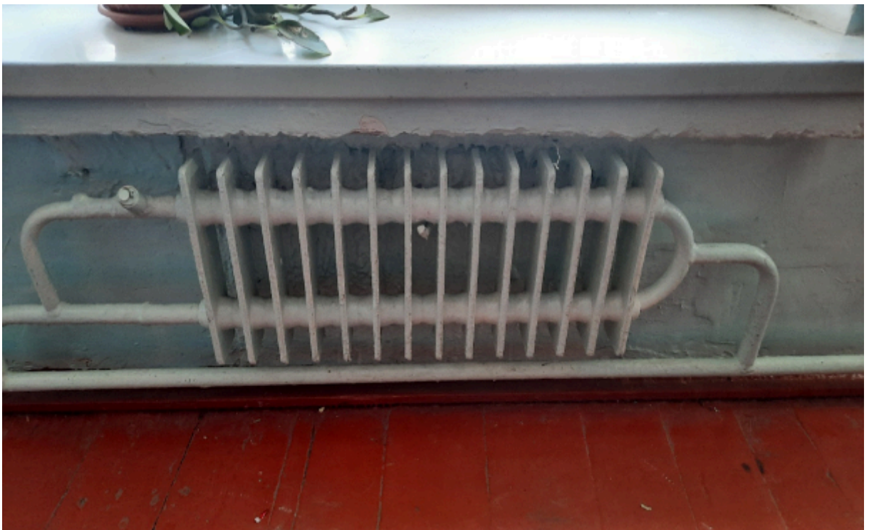
Photo 6. Type of plate radiators installed in building No. 2
